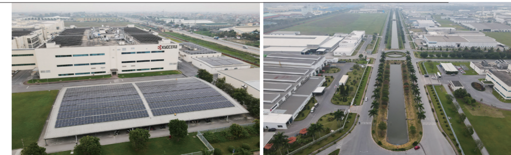
Solar panels being installed on factory roofs in TLIP to secure a stable supply of power and as an environmental measure (left). The vast site is even equipped with channels and retention basins to store rainwater for flood control (right). (Both photos are of TLIP II).
