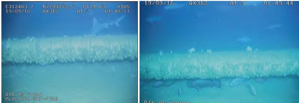
**Figure 5-2 Pipeline showing sandy substrate in the foreground, Pluto, depth = 179m**
