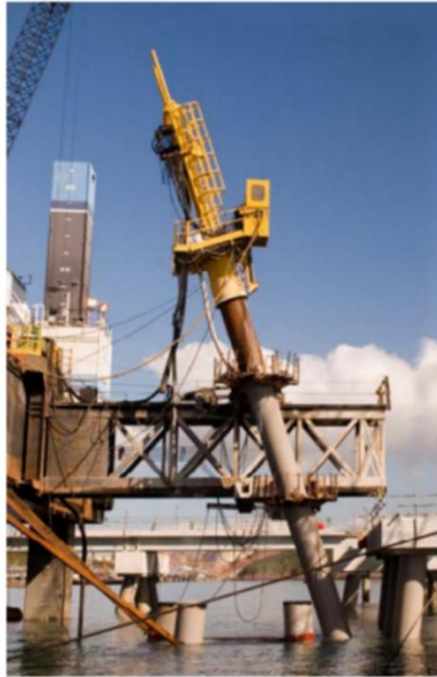
(a) Steel Pile Installation
