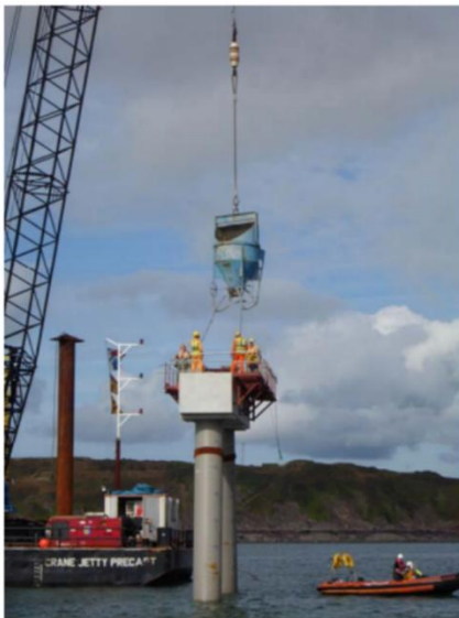
(c) In situ concreting
