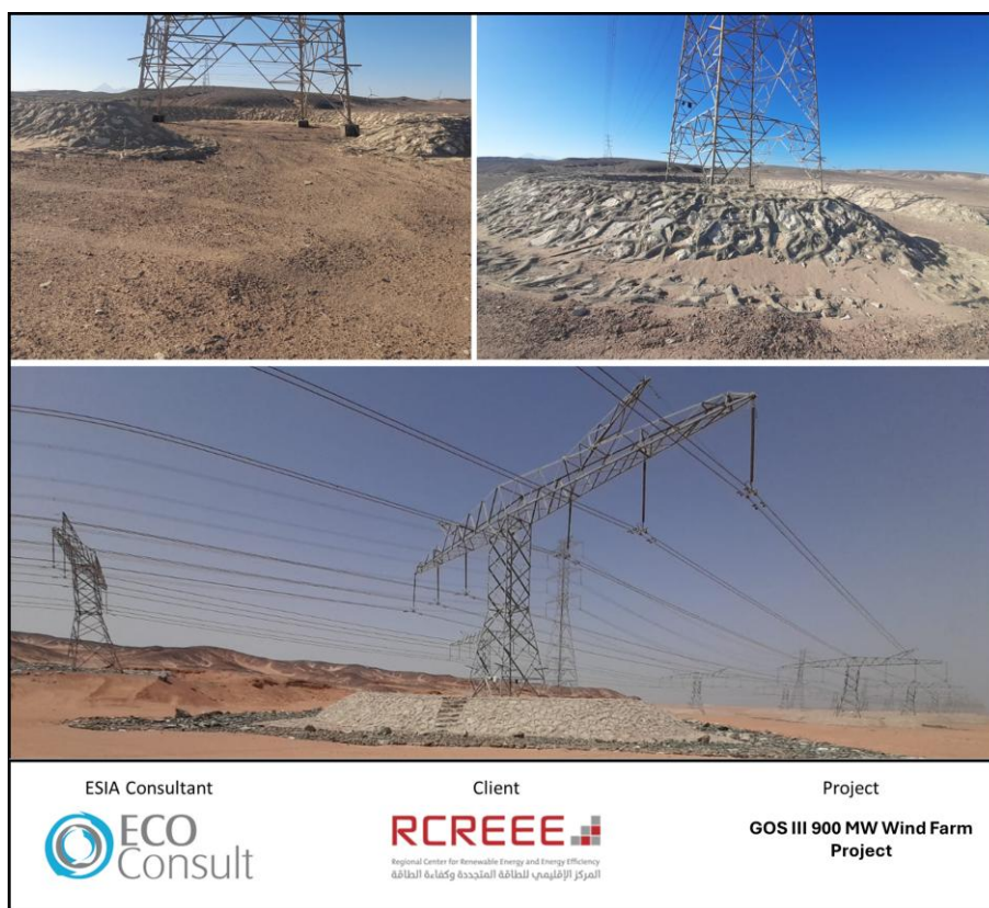
Figure 100: Simple Fences Applied to Protect the Base of Towers from Surface Flow Erosion
