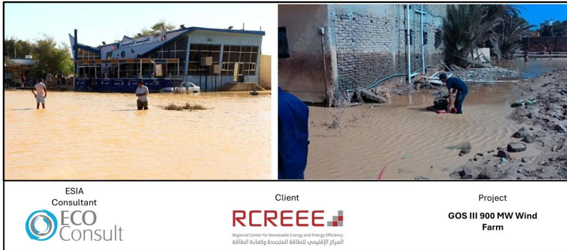
Figure 87: Observed Flood Damage in Ras Gharib During the October 2016 Storm Event
