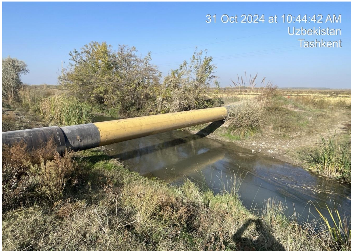
Figure 2-15 Gas Pipeline to the West of the Project Site
