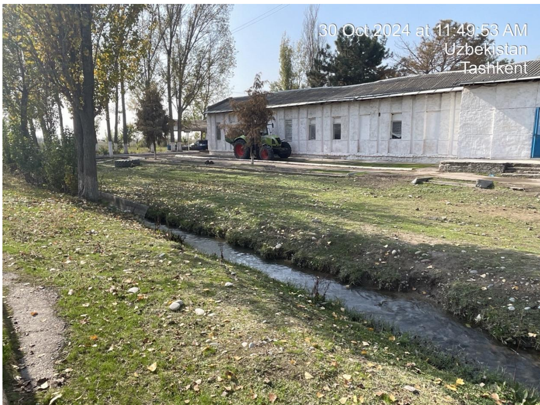
Figure 2-9 One of the Existing Buildings within Project Site
