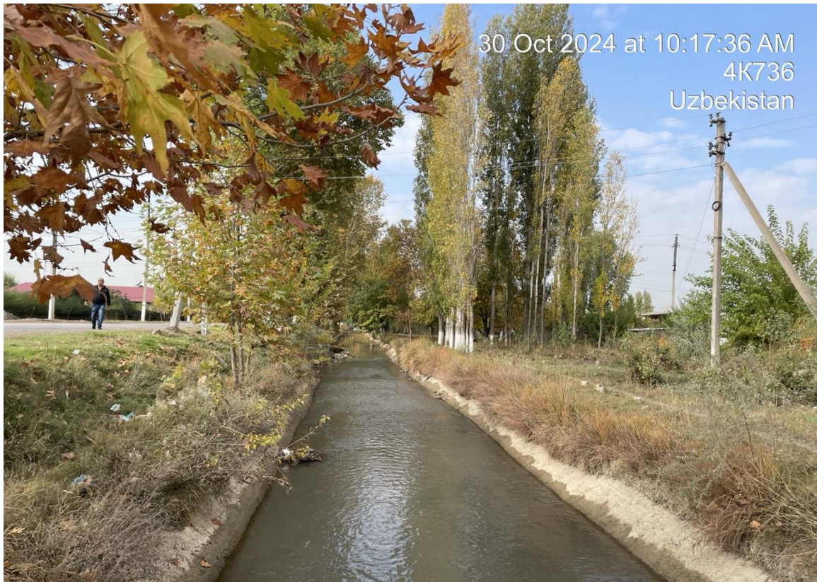
Figure 2-13 Canal to the South of the Project Site
