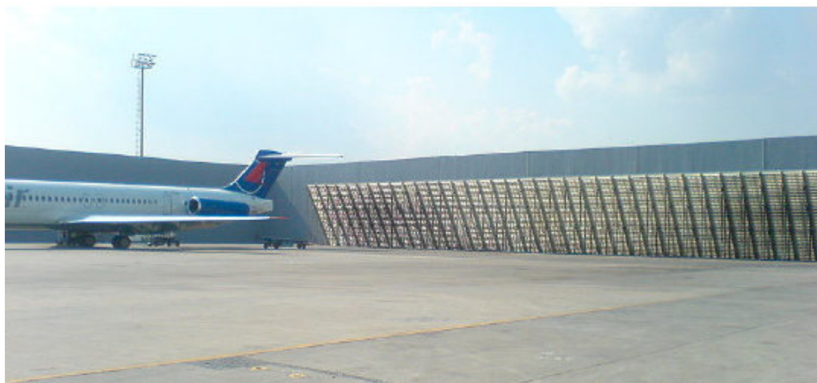
Figure 2-25 Example of an Engine Run-up Area at Istanbul Ataturk Airport
