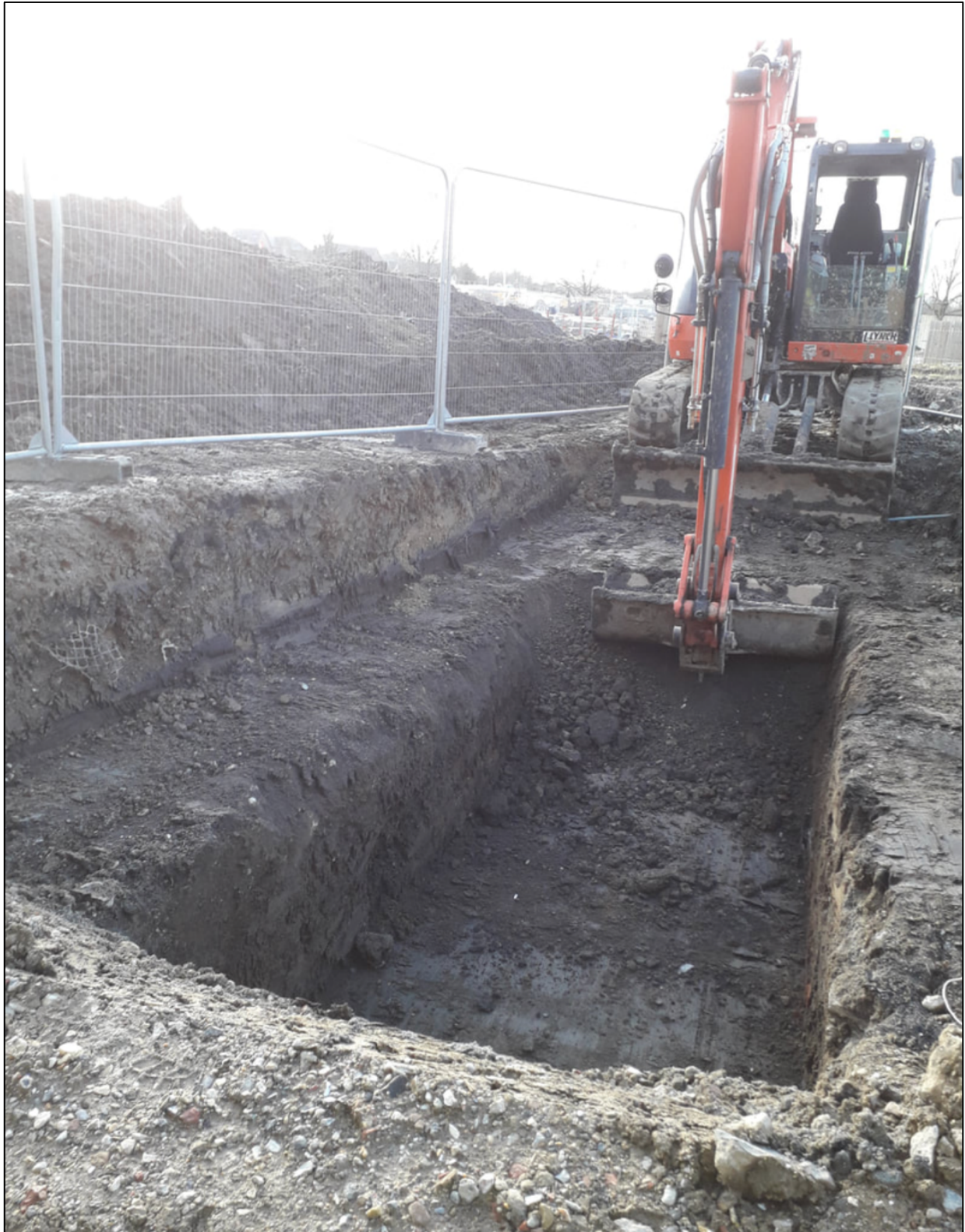
Figure 9. Example of two-stepped 2m deep trench (2m internal trench and 4m w external step) using mechanical 360 excavators fitted with a 2.0m-wide toothless ditching bucket.
