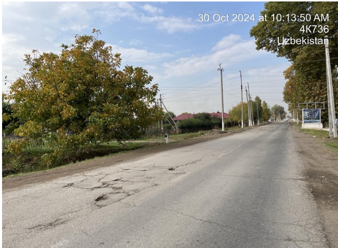
Existing Public Road to South of the Project Site
