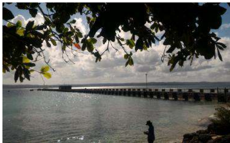
Gambar III-501 Jetty Depo BBM Pertamina
