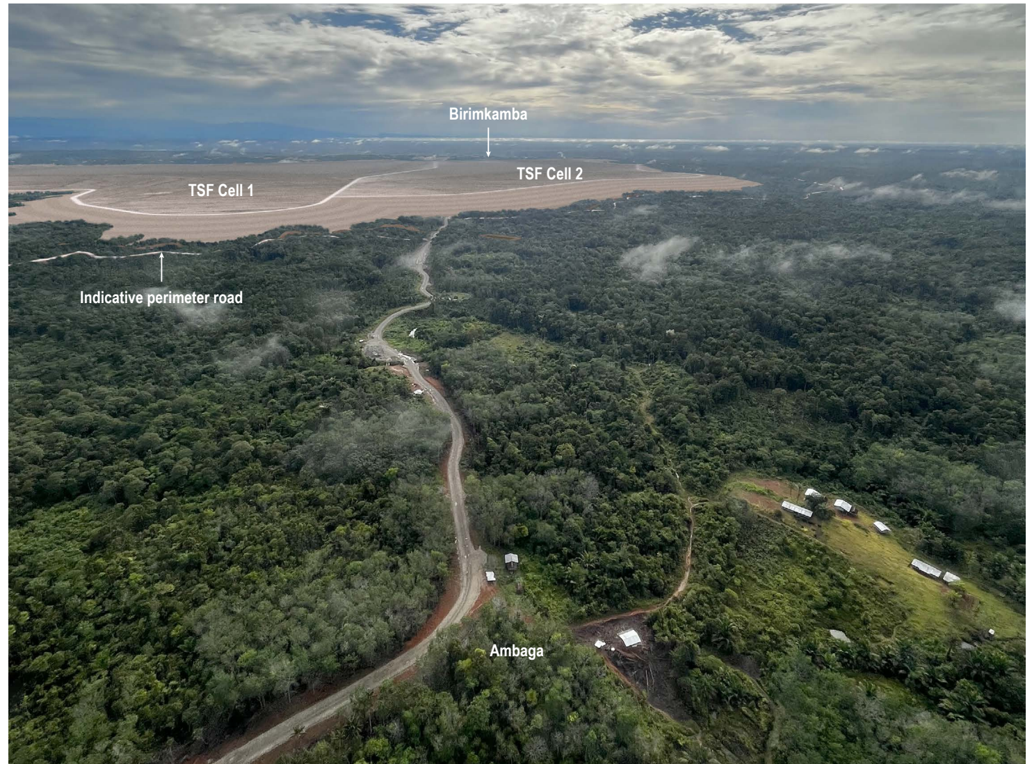
Aerial view at Ambaga looking east with the proposed TSF Cells 1 & 2
