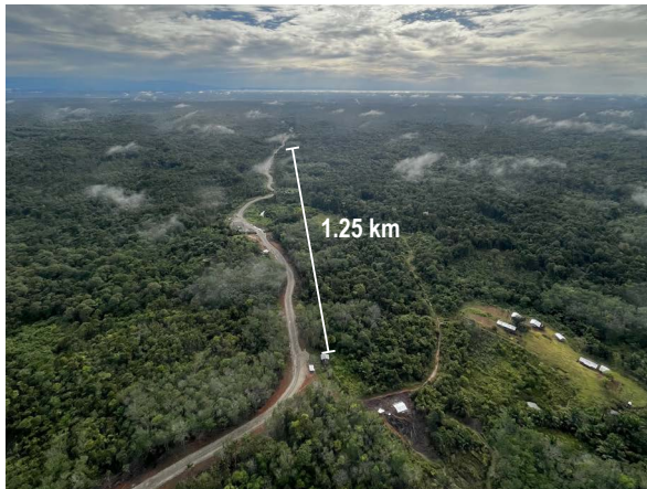
Aerial view at Ambaga looking east Existing Conditions
