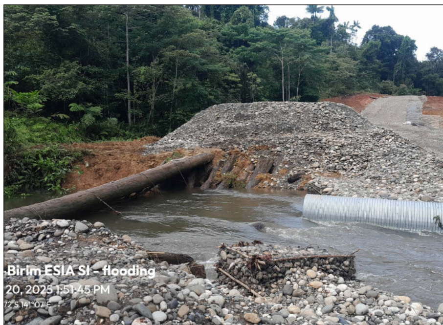
Plate 8.2 Roadway crossing over a perennial tributary
