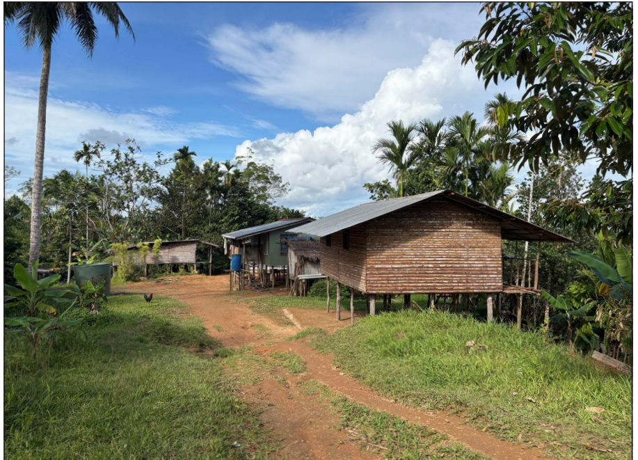
Plate 9.19 Example of a semi-permanent house
