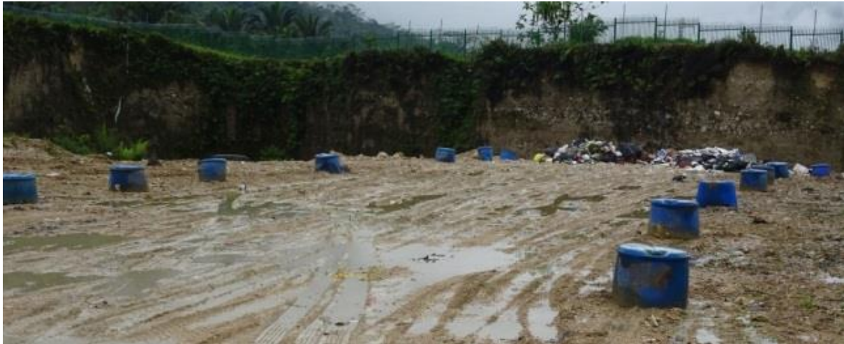
Figure 6 Tabubil Landfill Facility
