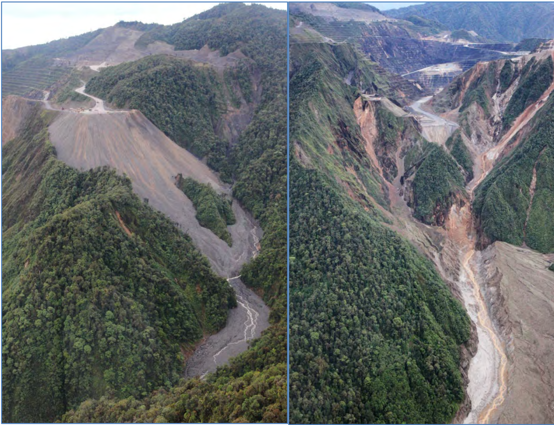
Figure 2: The new Northern Dump (left) showing a limited catchment area and limited toe losses. The Southern Dump (right) continues to have a high loss rate. Photos: January, 2014.
