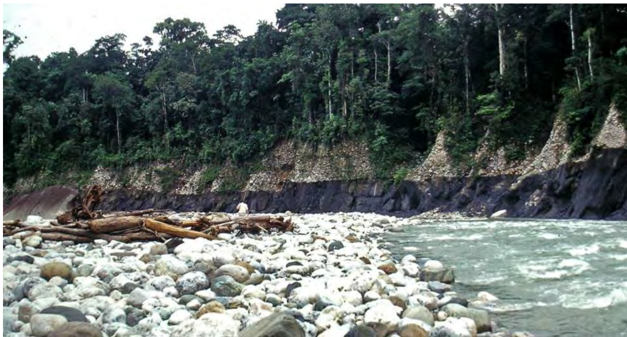
Figure 2-3. Former debris flow deposits on top of exposed bedrock in the upper reaches of the Middle Ok Tedi. Note the size of gravels in the riverbed which illustrate the transport capacity of the river. 1979 (pre-mine) photo.
