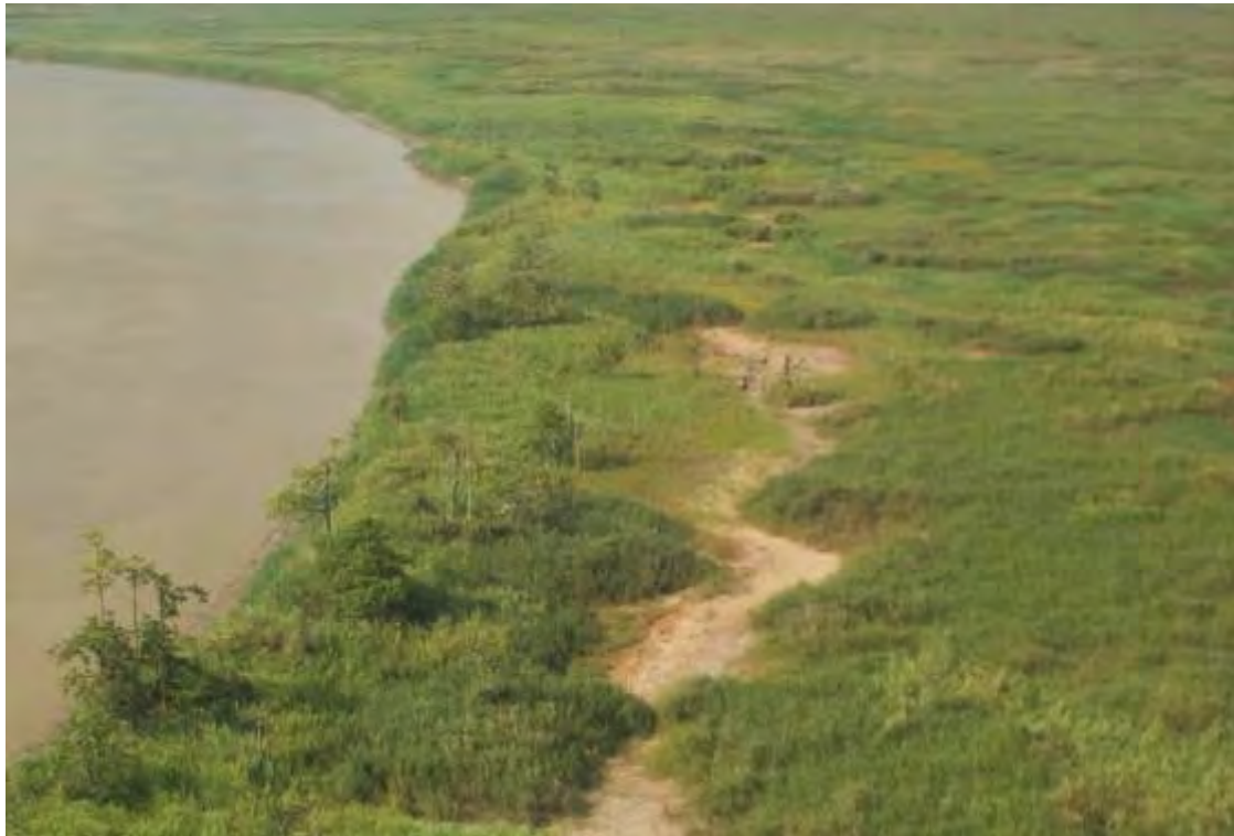
Figure 2-15. Vegetation impact on levee backslope due to high acidity water seepage. Photo from 2006, site is now NAF.
