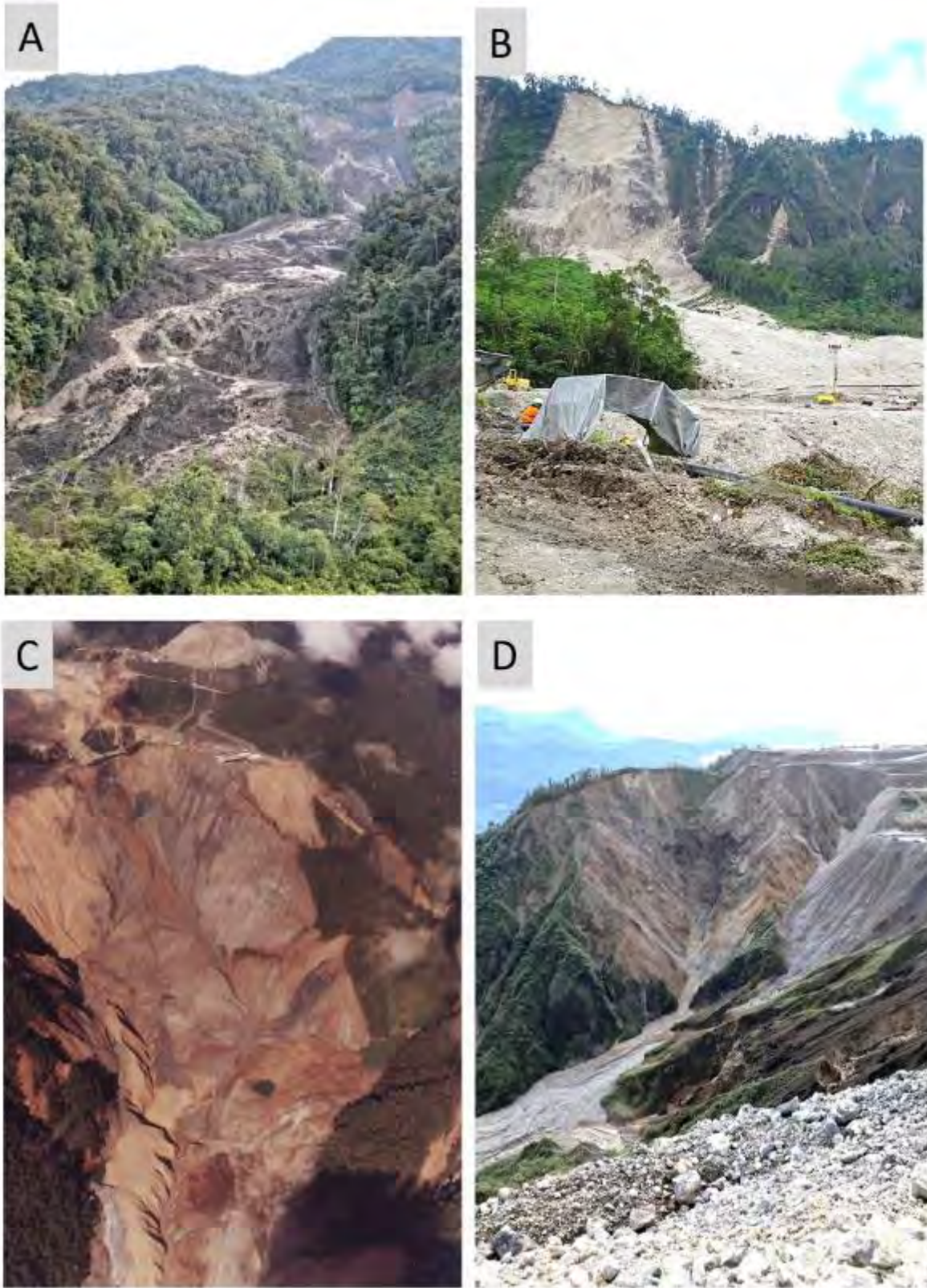
Figure 3-5. Significant landslides in the mine area. (A) a mudslide from weathered material on the Ok Kam (B) a rock avalanche from probable old Hindenburg Wall landslide debris flow deposits north of Tabubil which cut the mine access road and caused damage to pipelines. (C) the massive 1989 Vancouver Ridge slope failure which caused waste rock dumping to shift from the north side of the mine to Harvey Creek on the south side. (D) the ongoing New York Ridge rock avalanche.
