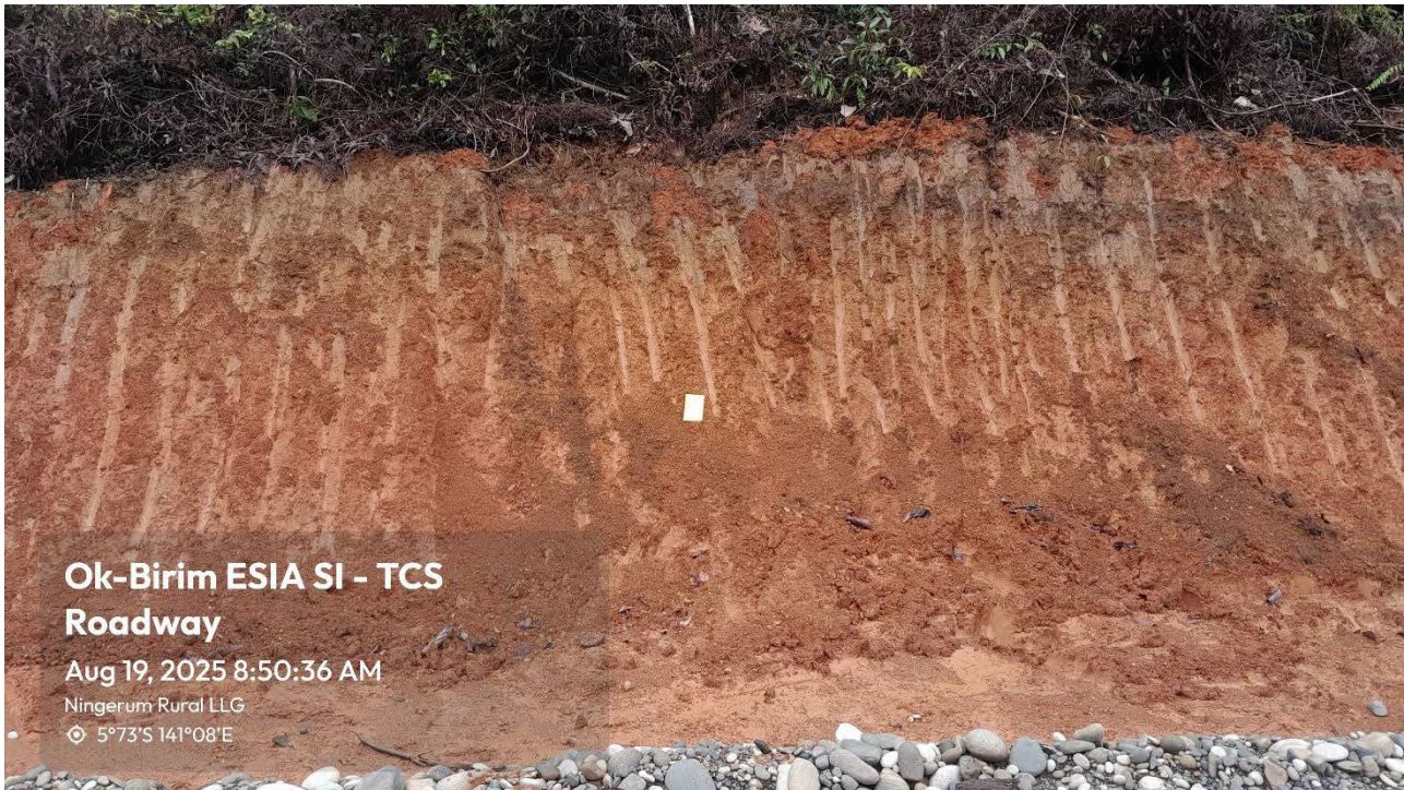
Figure 5.8 Road cutting exposure of the ridgeline soil profile.
