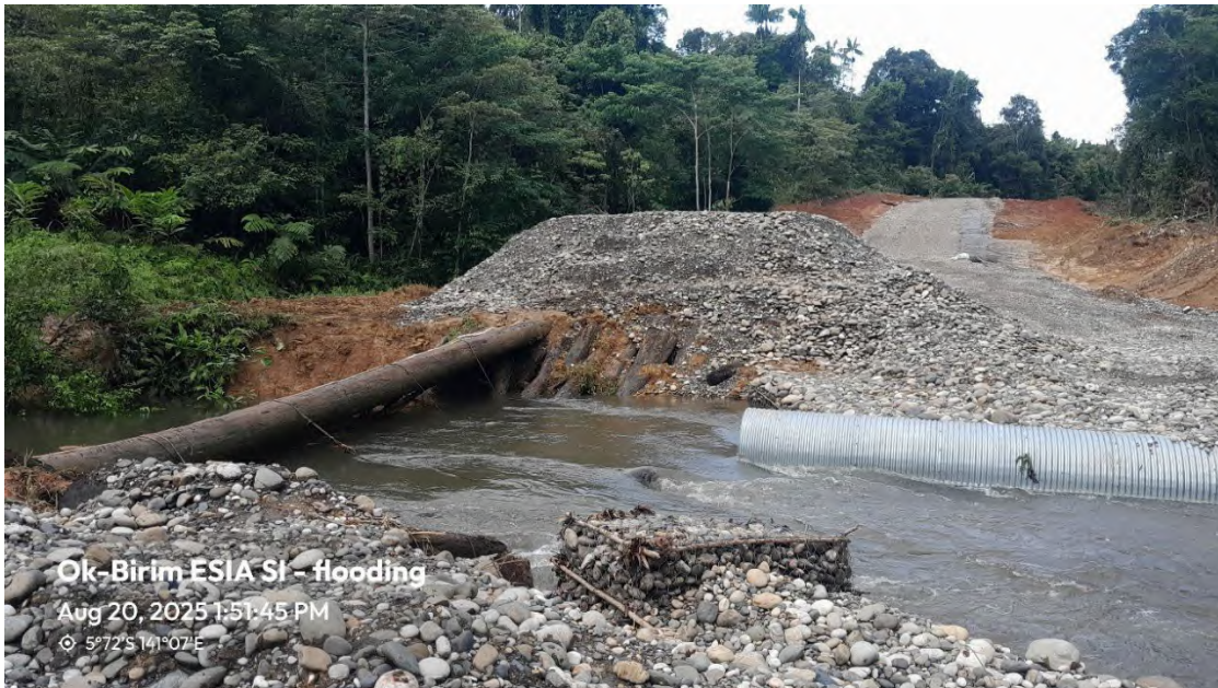
Figure 5.5 Roadway crossing at one of the permanent tributaries near KCB25-TP7008.
