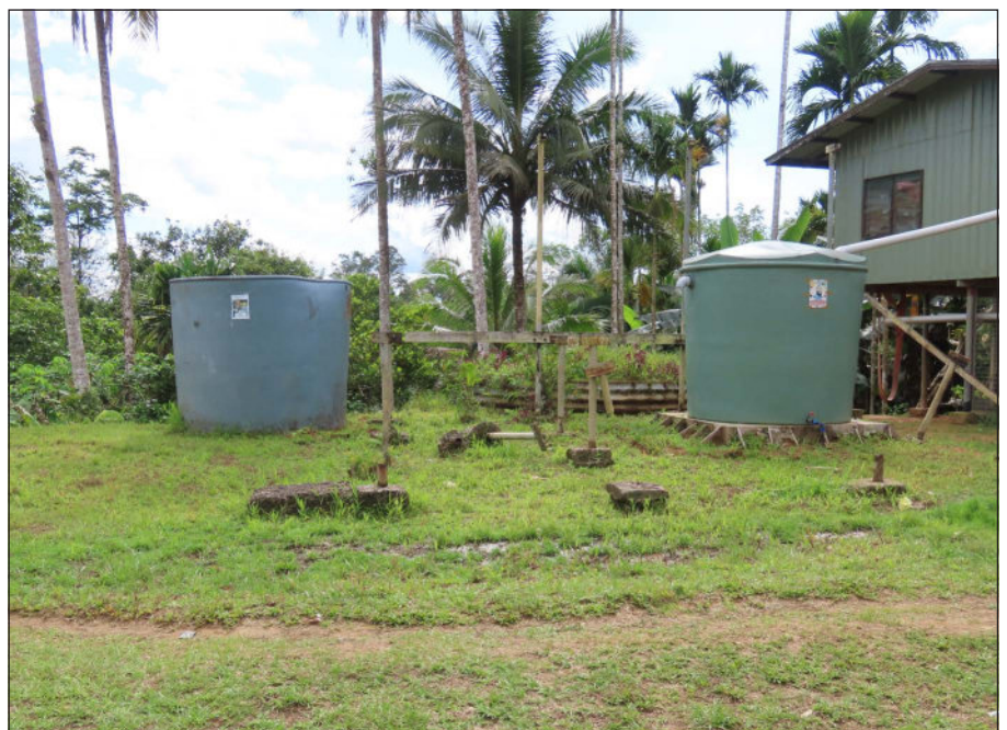
Plate 6.39 Rainwater tanks, Birimkamba village
