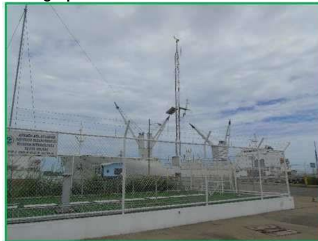
Photograph 2: Puerto Bolívar Weather Station
