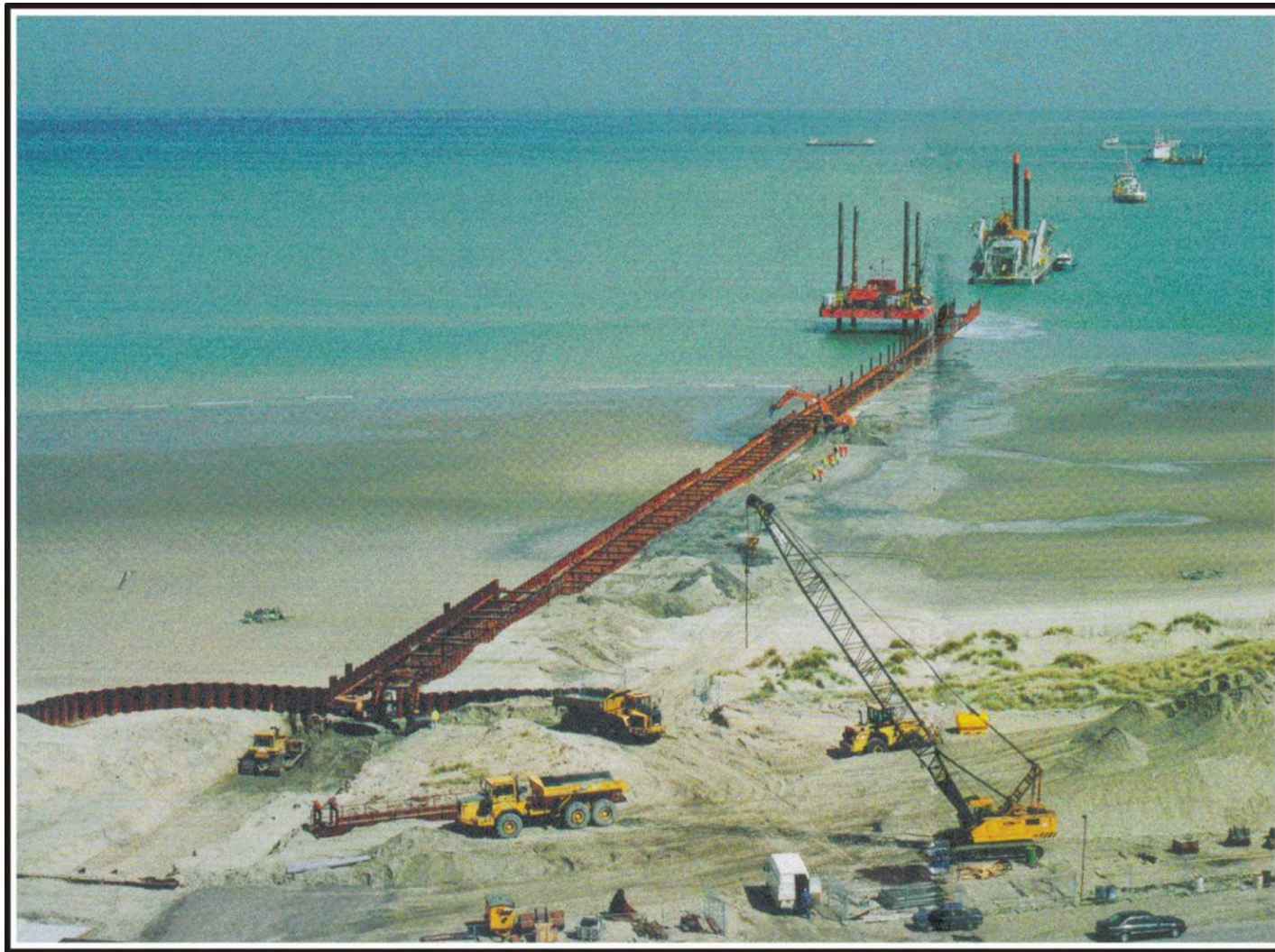
Figure I-16 Conceptual Trenching and Shore-pull Activity
