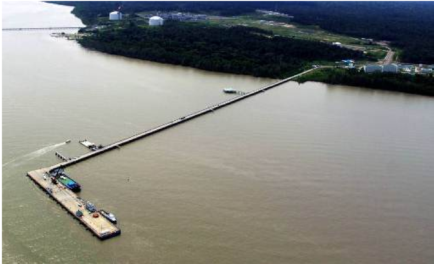
Figure I-55 Existing Combo Dock
