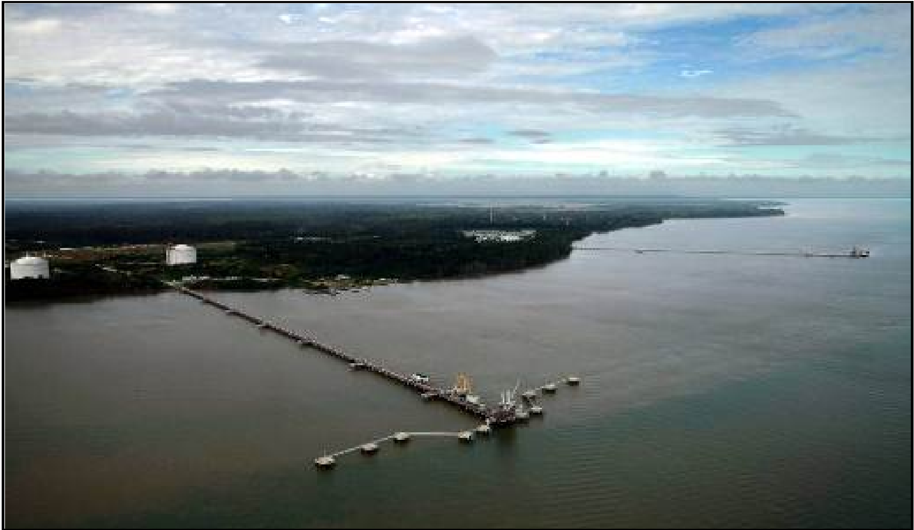
Figure I-40 Existing Marine Facilities in Tangguh LNG
