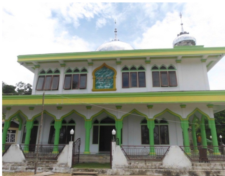
Figure II-218 Mosque in Arguni Village, Kokas District
