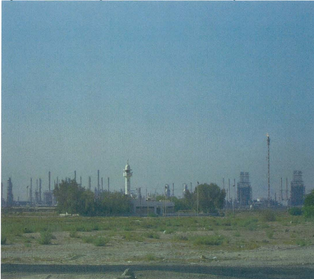
Figure 14C: View looking north from south of MAB refinery
