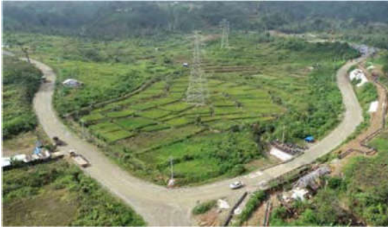
PLN Transmission Line - Associated Facility
