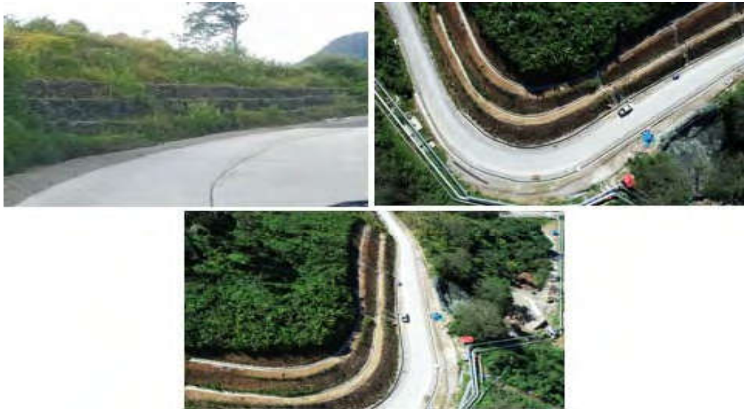
Dust Emmission Mitigation by Road Pavement
