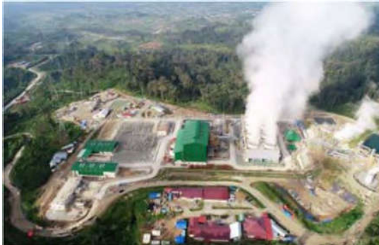
Power Plant Area
