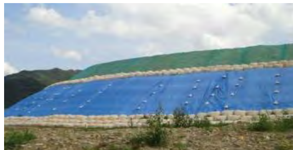
[Sample of Covering]
