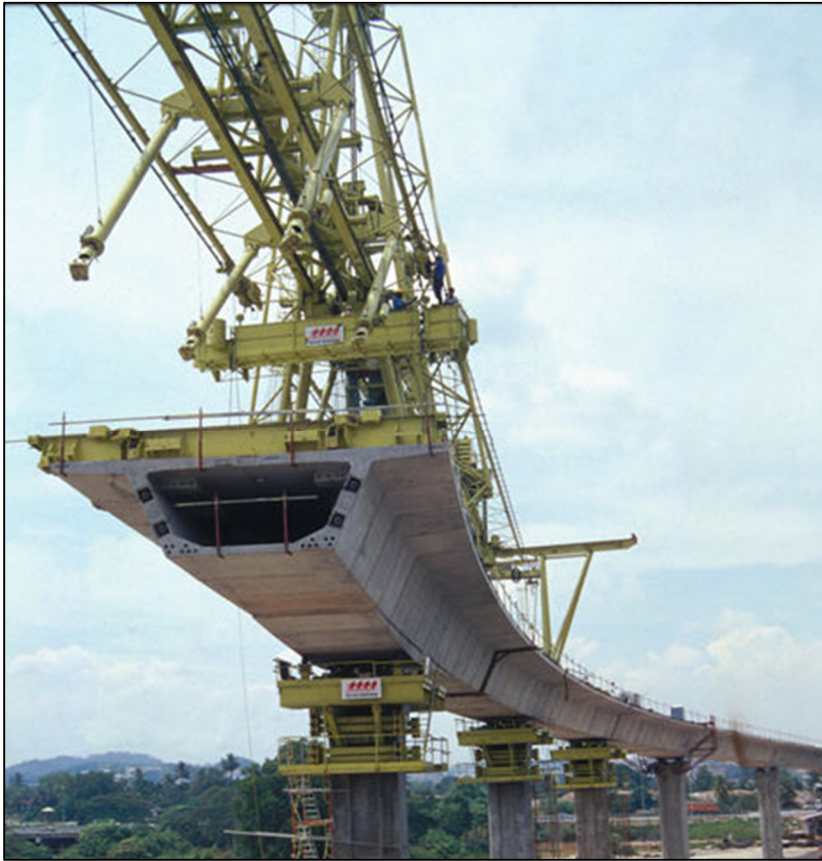
Figure 7: Balanced Cantilever, STAR Light Rail, Kuala Lumpur, Malaysia ( Photo courtesy Arup )
