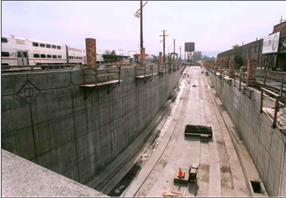
Figure 10: Trench Diridon Tunnels, San Jose, CA
