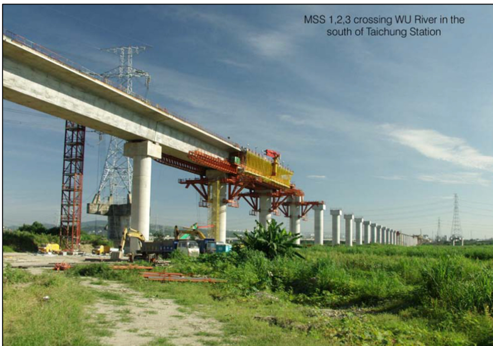
Figure 9: MSS Moving Forward to the Next Span, Bent Construction Well Advanced of the Girder Placement, Taiwan High-Speed Rail, ROC (Photo courtesy of THSRC)
