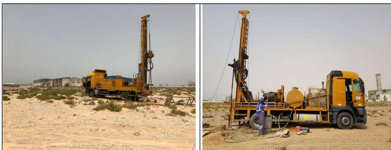
Figure 4: General photograph during drilling of boreholes
