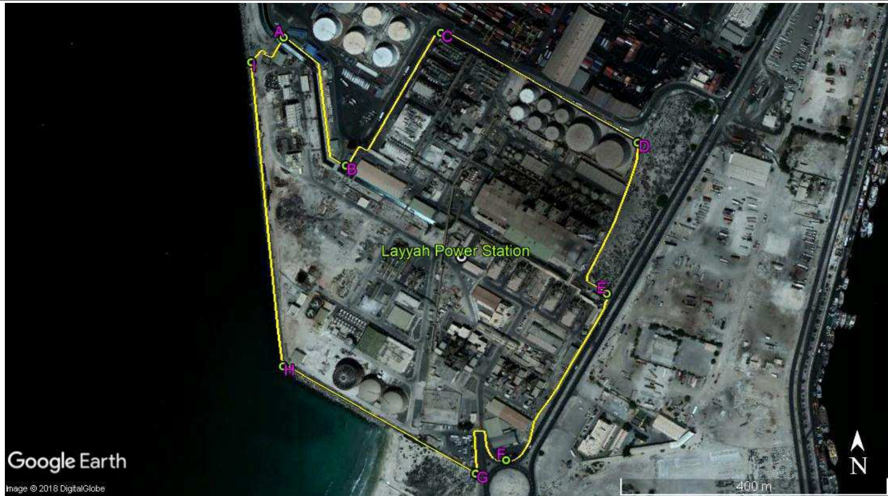
Figure 2 - Google Image showing the project site
