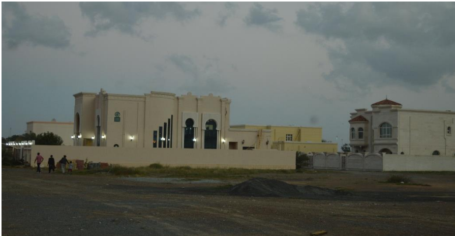
Figure 4-8: Example of residential houses
