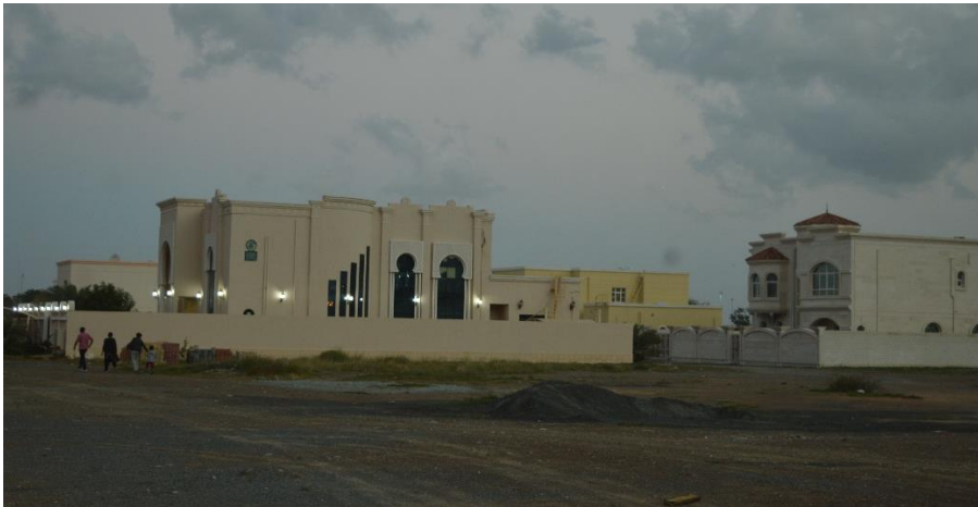
Figure 5-8: Example of residential houses (refer to P7 in Figure 5-10)
