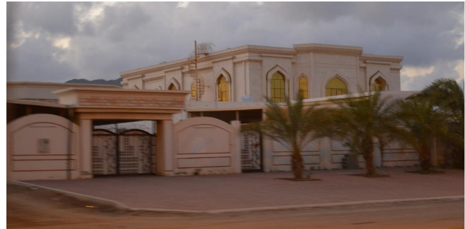
Figure 5-9: Example of a residential house (refer to P8 in Figure 5-10)
