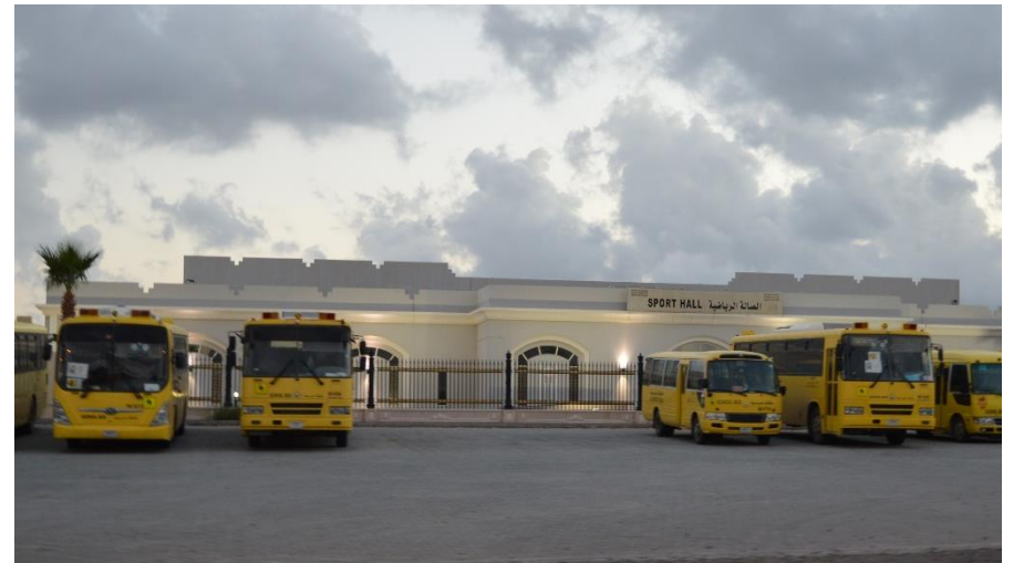
Figure 5-5: Sport Hall of Alnoman bin Almoqren School and Merbah Secondary School for Girls (refer to P4 in Figure 5-10)
