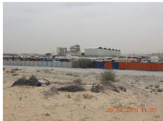
View of concrete producing plant(s) along western site boundary (facing west)
