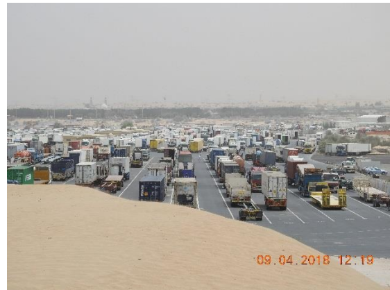
View of existing parking area over asphalt pavement (facing east from edge of site)
