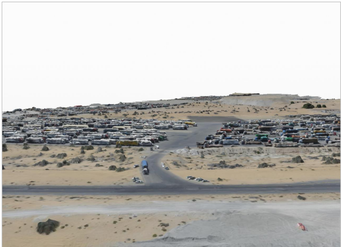
Figure 5-42 View of the existing site conditions
