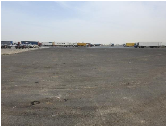
View of millings driving surface, asphalt paved area with truck parking beyond (facing north)
