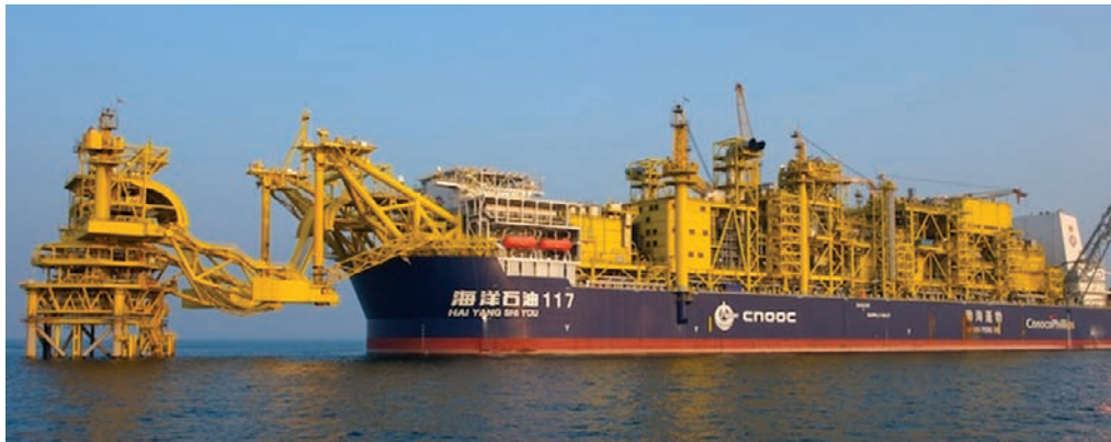
Figure 4-6: Example FPSO facility
