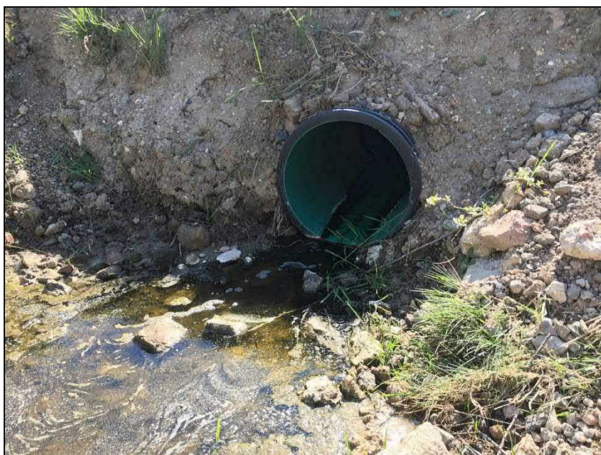
Figure 2: Culvert beneath track crossing at spot check 1 (looking upstream)
