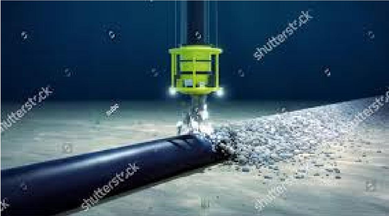
The placement of specifically graded rock on a surface laid cable to protect against external threats such as fishing and dragged non holding anchors, is a well-established protection method in the North Sea area.
