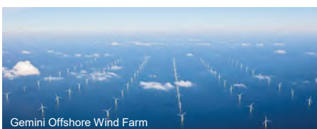
Gemini Offshore Wind Farm
