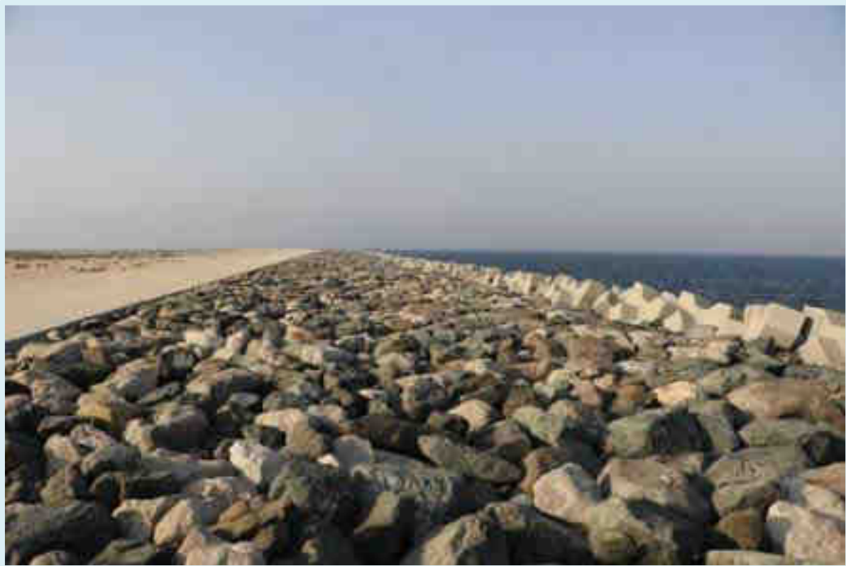
Plates 7 & 8: Rock armouring revetments
