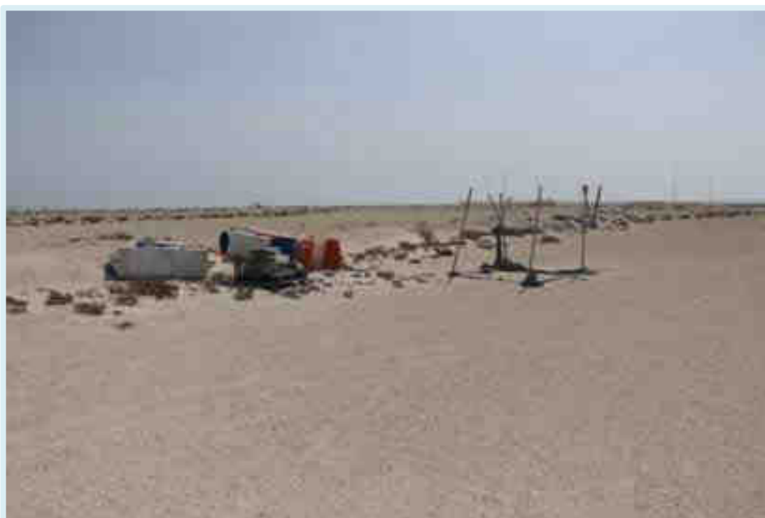
Plate 19: Construction materials at the northern end of the site
