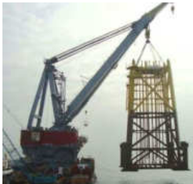
Levage de la structure (source : www.heavyliftspecialist.com )
