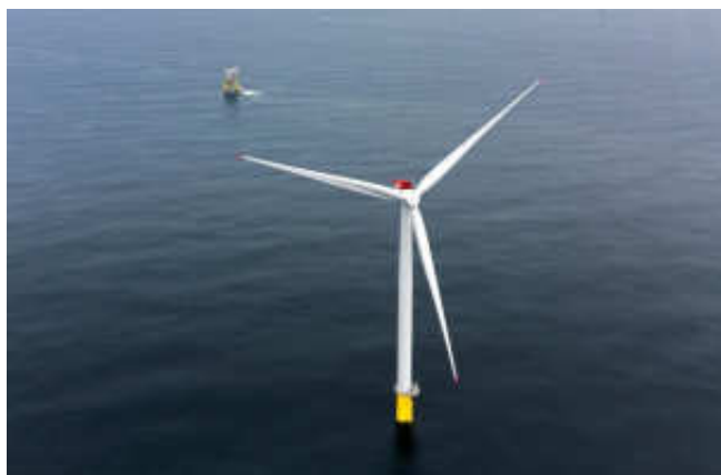
Source : Siemens-Gamesa Renewable Energy, 2017
