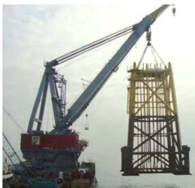
Levage de la structure (www.heavyliftspecialist.com)
