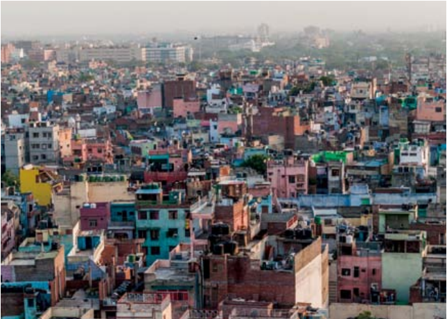
Delhi, India: Buildings under construction
