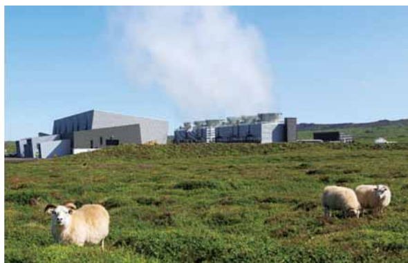
Geothermal power project in Iceland in which Japanese companies are participating
