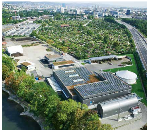
Waste treatment plant in Sweden
