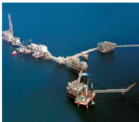
Abu Dhabi offshore oil field project (provided by INPEX)
