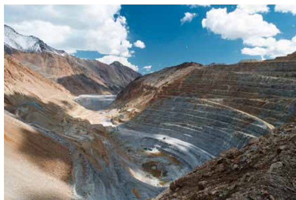
Los Pelambres copper mine expansion project in Chile (provided by Antofagasta Minerals S.A.)
