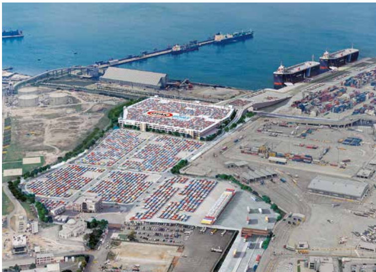
A car logistics terminal operation project in Turkey
