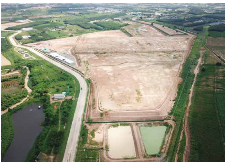
Gulf PD Natural Gas-Fired Combined Cycle Power Plant Project
