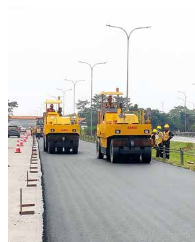
Paving works with recycled asphalt in Indonesia
