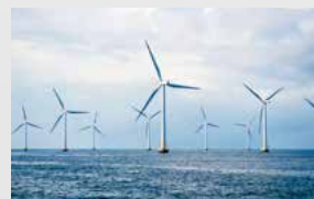
Moray East offshore wind power generation project in the UK
