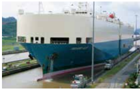
Panama Canal Expansion Project
