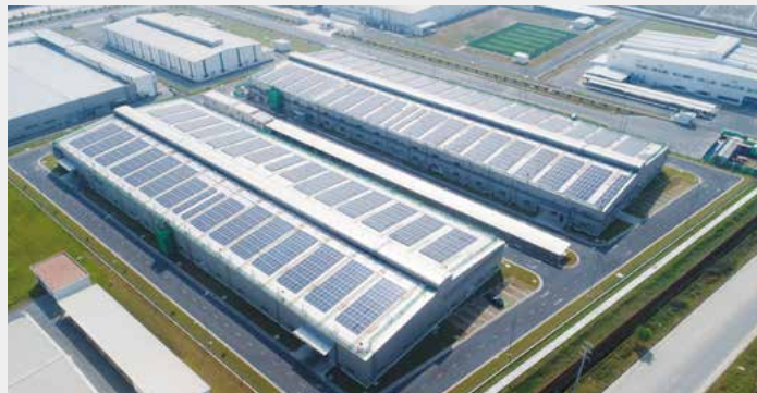
Rooftop solar power generation project of Thang Long Industrial Park II
