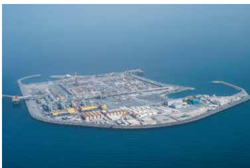
Oil and gas field production facilities
