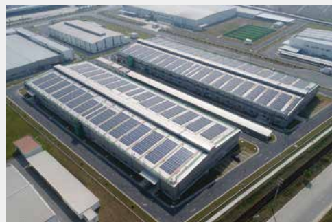
Expansion project of Thang Long Industrial Park II
