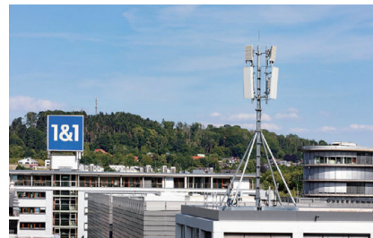
JBIC is supporting the overseas expansion of Japanese companies aimed at developing reliable infrastructure in the digital sector.
