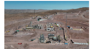
(Source : Nittetsu Mining) Arqueros Copper Mine construction site.
