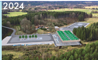
③ Geothermal power generation and district heat supply project in Germany Source: website of Chubu Electric Power Co., Inc.
