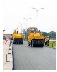
Paving works with recycled asphalt in Indonesia
