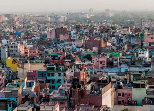
Delhi, India: Buildings under construction
