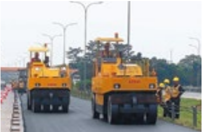
Paving works with recycled asphalt in Indonesia
