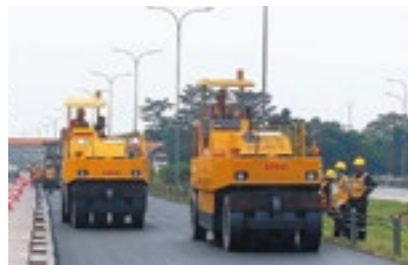
Paving works with recycled asphalt in Indonesia
