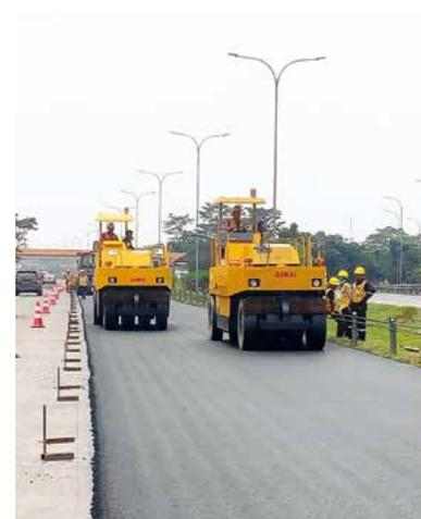
Paving works with recycled asphalt in Indonesia
