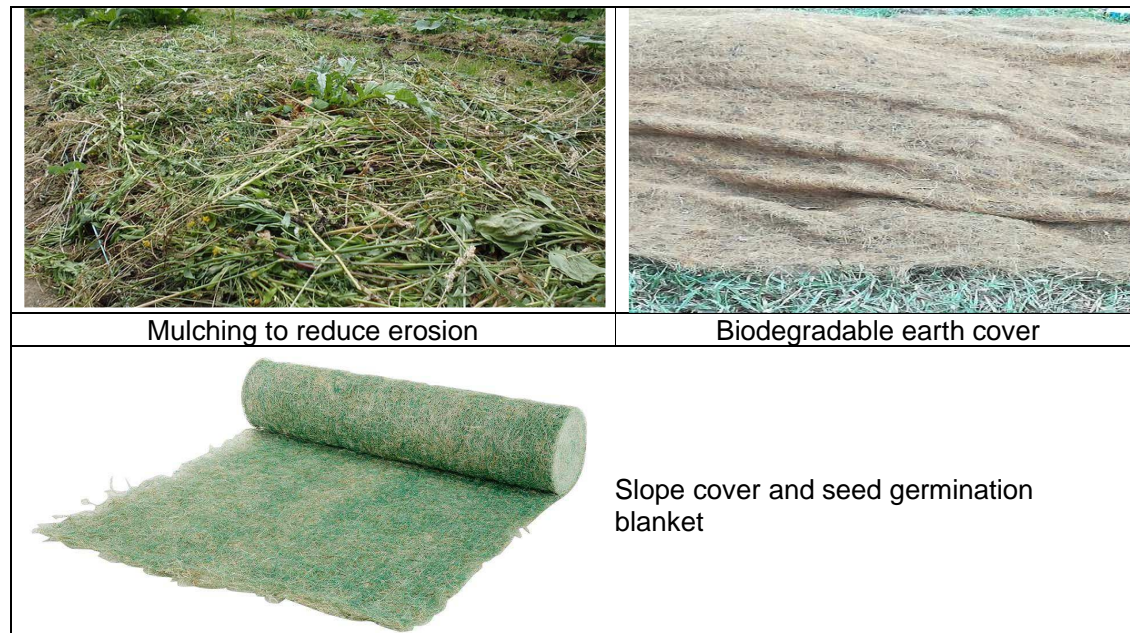
Figure 8.2(2): Earth Covers by mulching or biodegradable covers
