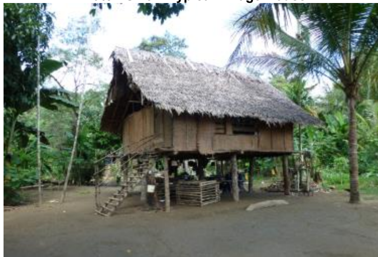
Plate ES2.3 – Typical Village House
